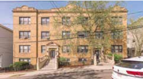
The majority of our existing housing stock in consolidated neighborhoods are NOAHs. Non-profit developers like TND have projects like Chelsea Legacy that renovates and repairs these buildings and extend their affordability.
