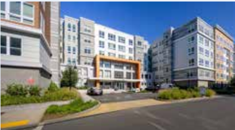
Vero Apartments: Large, 692-unit mid-rise luxury residential community developed by Fairfield Residential. It was permitted in 2015 prior to the Inclusionary Zoning Ordinance, so only 3% of units (21 units) are affordable at 80% AMI.
